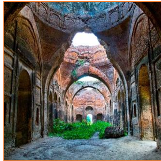
Phuta Mosque, Murshidabad
